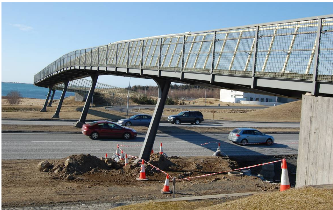
Figure 11. Walking bridge across Kringlumýrarbraut. (Location 1)
