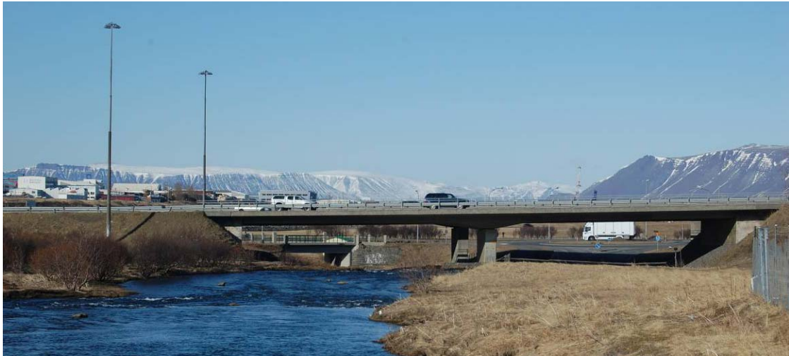
Figure 12. Picture of the Vesturlandvegur bridge over Elliðará. (Location 2)
