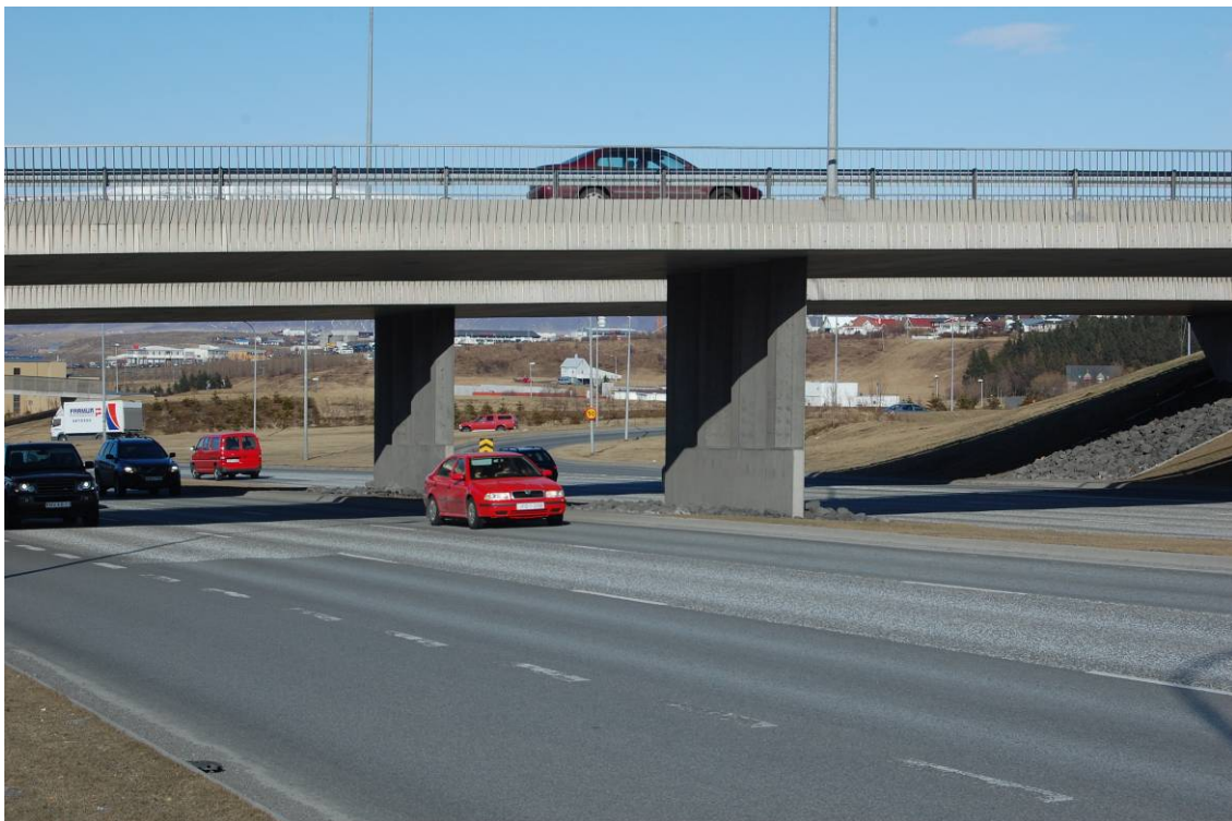
Figure 15. Picture of the Höfðabakki aqueduct over Reykjanesbraut. (Location 3)
